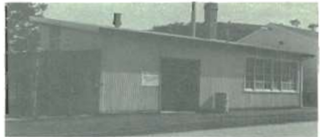
The now disused welding shop which dates from before the establishment of the college. Part of the original Robert Campbell property which was established in the 1930s. It contains a forge and was originally used as a Farriers shop.
